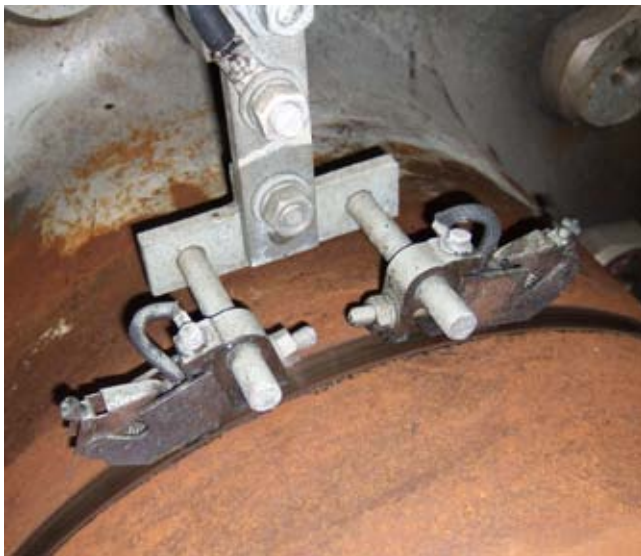
No seperate slip ring installed
