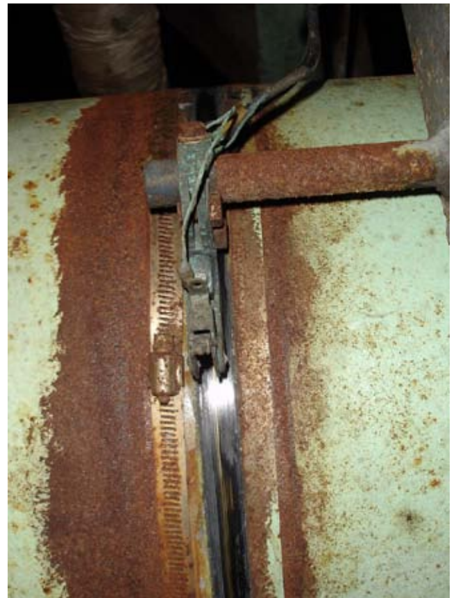
Brushes and cables that do not meet MAN specifications
